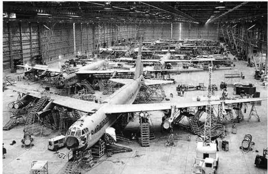
The aircraft maintenance hangar, here and above, at the San Antonio Air Materiel Area at Kelly could house 13 B-52s at once. The same hangar was later used to overhaul eight C-5s at a time. By then, SAAMA had become the San Antonio Air Logistics Center.
