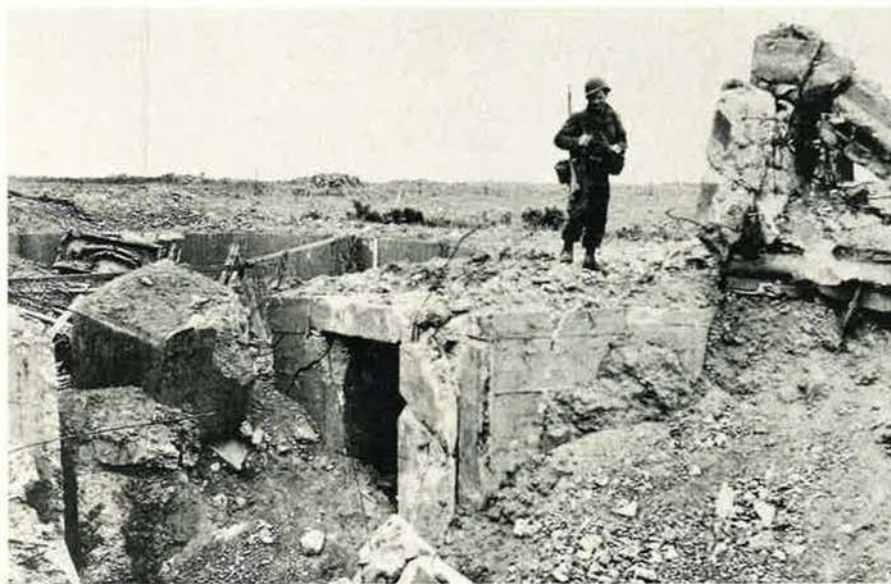
Pulverized from above. A US soldier surveys bomber damage to a German gun emplacement in France. Much of the Nazis' vaunted "Atlantic Wall" looked like this after heavy and medium bombers did their work preparatory to D-Day.
