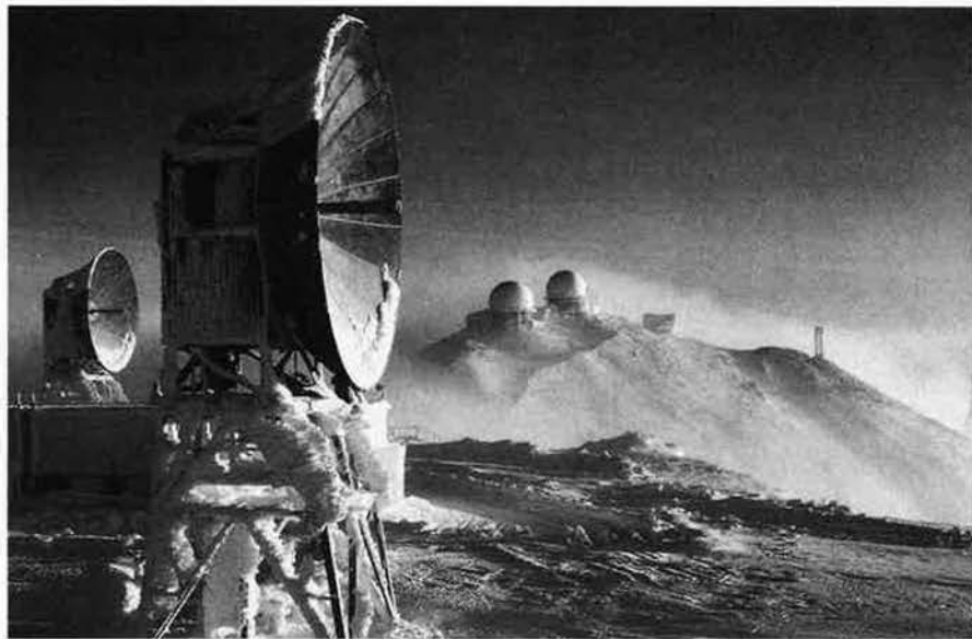
On the ground in the late 1950s, air defense in the far north included radars on the DEW Line, amid windswept peaks on the frozen landscape. Construction of the DEW Line was the largest building project in the Arctic.
