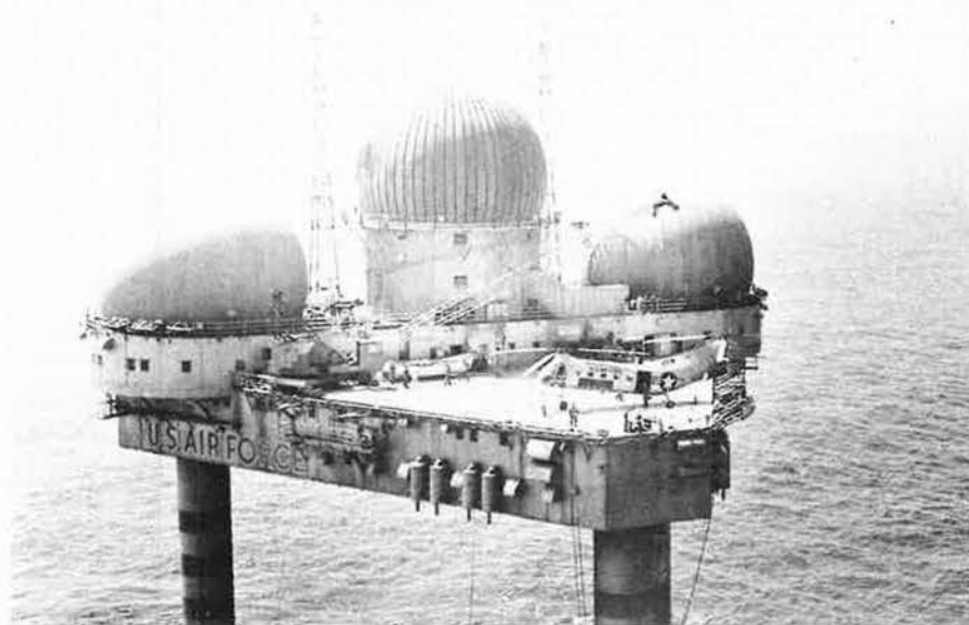
A more radical idea for early warning: Texas Towers, named for their resemblance to oil-drilling platforms. The radar stations rose from the sea, off the northeast coast of the US. This is TT-3, located south of Nantucket, Mass. The last of the towers was decommissioned in 1963.
