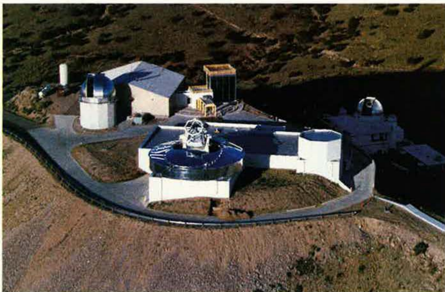
Correcting atmospheric optical distortions was key to making the ABL feasible. Deformable mirrors on this telescope at Kirtland AFB, N.M., paved the way for the ABL. The telescope can also image orbiting spacecraft with great clarity.
