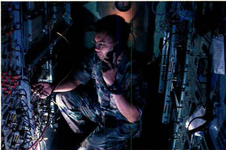
During a recent Cobra Gold '99 at Korat AB, Thailand, TSgt. Michael Amposta, 613th Air Communication Squadron, Andersen AFB, Guam, helps link ground terminals to satellites in space. The annual exercise improves US and Thai combat readiness and interoperability.
