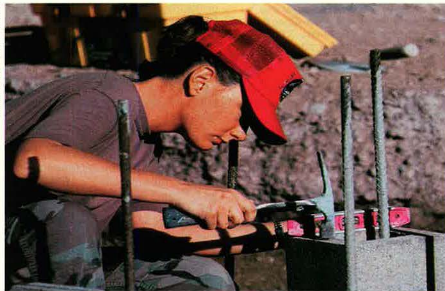
Members of the 823d RED HORSE Squadron, Hurlburt Field, Fla., participated in a US Southern Command exercise on St. Kitts-Nevis. At top, the engineers place restraining walls for a building at Camp Springfield, St. Kitts, while (above) A1C Christine Hensley levels out a block during construction of an operations center for the St. Kitts Defense Force.
