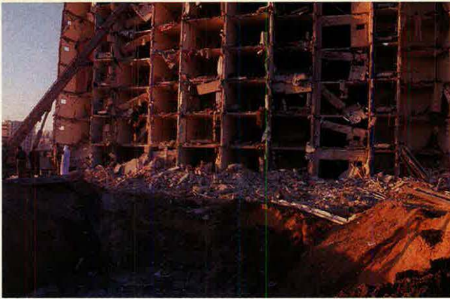
Although many new security measures had been implemented at the Khobar Towers high rise, it was not enough to deal with a truck bomb that detonated with the equivalent of 20,000 pounds of explosives.
