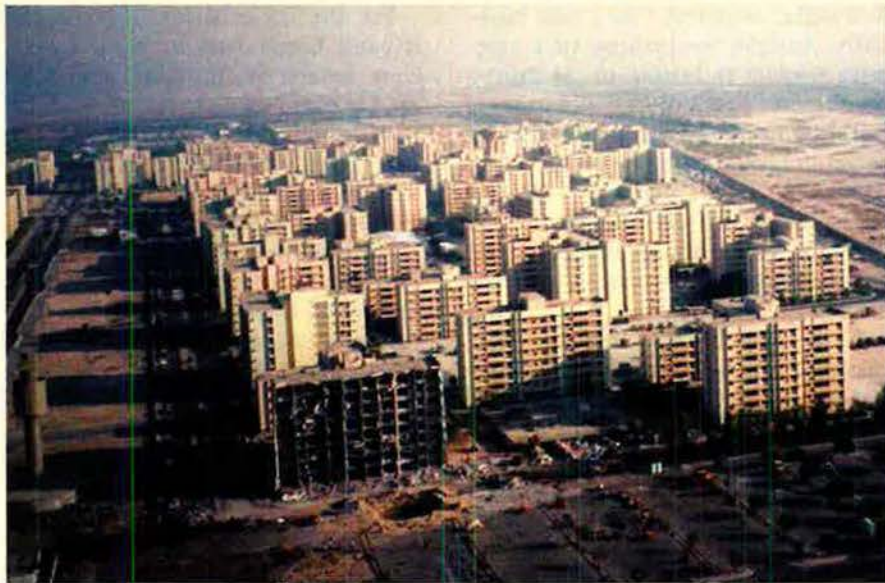
This photo of the Khobar Towers complex in Dhahran, Saudi Arabia, clearly shows the devastation of Building 131 by the bomb that exploded June 25, 1996, killing 19 Americans. The building did not collapse because it was built with prefabricated cubicles bolted together.
