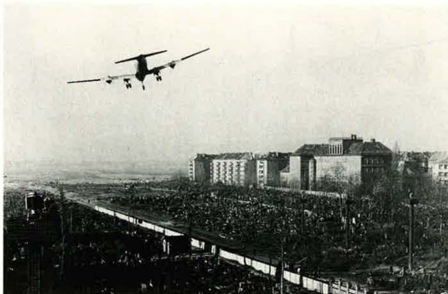
The often poor visibility at Tempelhof led the Air Force to install a high-intensity lighting system. Two parallel rows of 20 lights each mark the 3,000-foot approach as yet another C-54 makes its landing.
