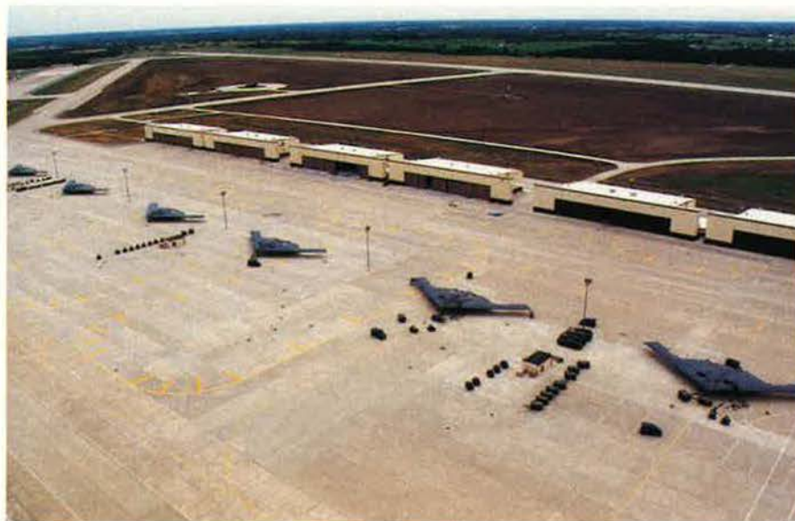
Behind six B-2s on the ramp at Whiteman AFB, Mo., are special hangars—with maintenance ports and hookups positioned to mate with the bomber. USAF is also acquiring some portable shelters in which personnel can carry out touch-ups to maintain the B-2's stealthy coating at a forward base.
