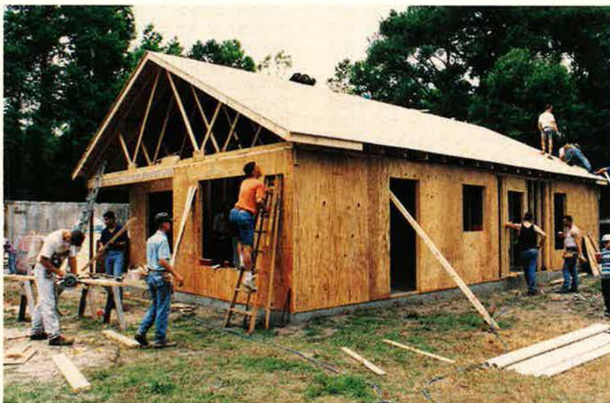
Members of the 437th Civil Engineer Squadron at Charleston AFB, S.C., showed their expertise by constructing this home in only three days as part of a "blitz build" project with the local Habitat for Humanity group.
