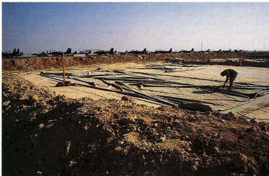
Prospective bases for an AEF must have ready access to water and fuel, and prepositioned equipment, such as fuel bladders, helps to reduce the amount of equipment that AEFs must carry with them.
