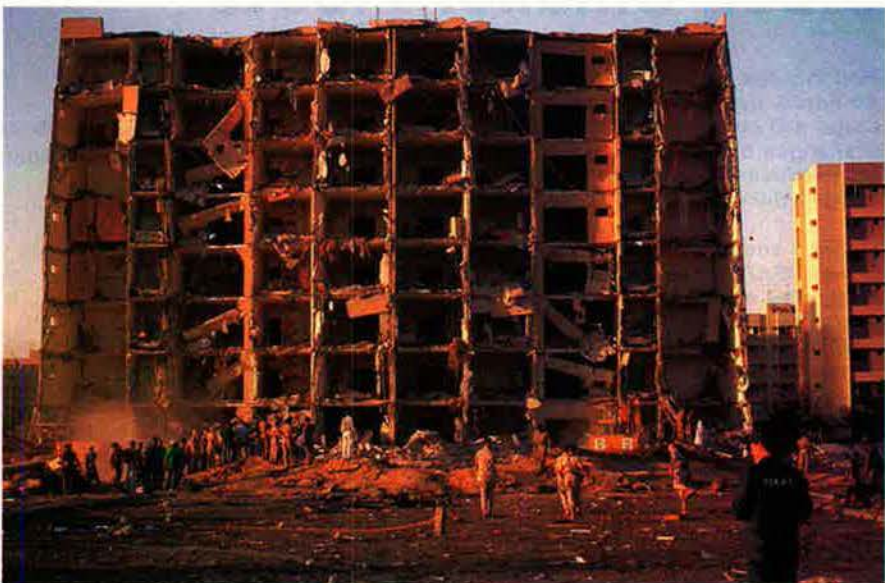
US and Saudi military personnel survey the damage to Khobar Towers from the June 25 truck bomb that exploded outside the security fence, about 100 feet from the facility on King Abdul-Aziz AB, Saudi Arabia. Since the attack, workers constructed a new boundary of concrete barriers about 400 feet from the US forces' residential complex.
