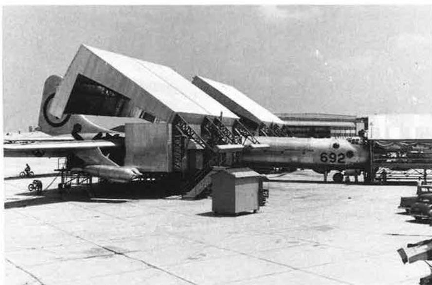
With its 160-foot length and forty-six-foot height, the B-36 was too large for most hangars, so USAF was forced to devise other solutions to allow mechanics to work on the bomber and yet be sheltered from the elements.
