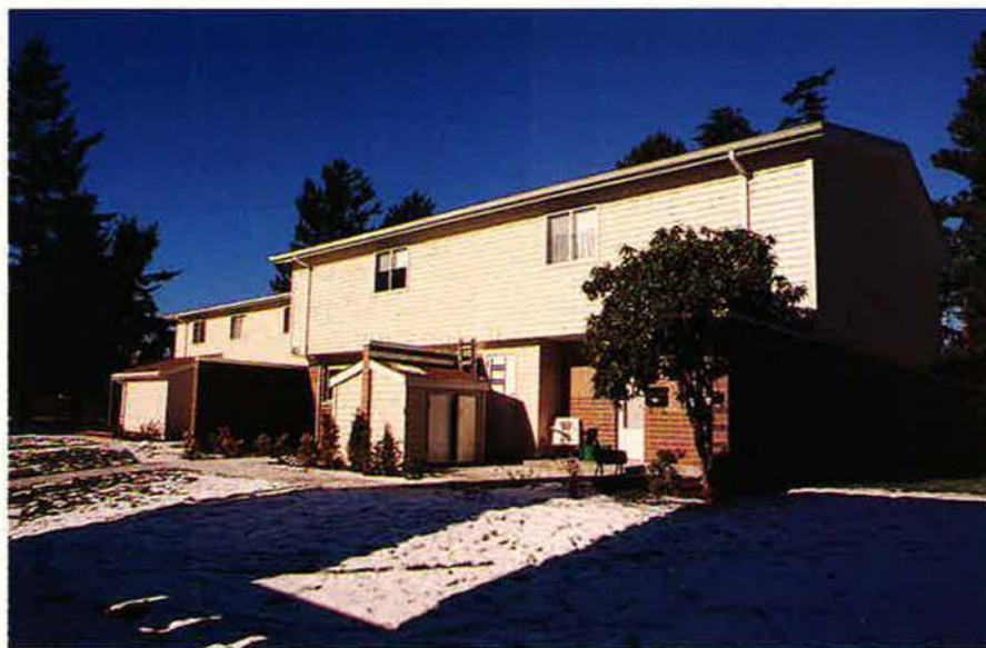
USAF has renovated about 23,000 family homes since 1988. These 1960s-era townhouses, home to enlisted members and their families at McChord, were among the housing units renovated in 1995.
