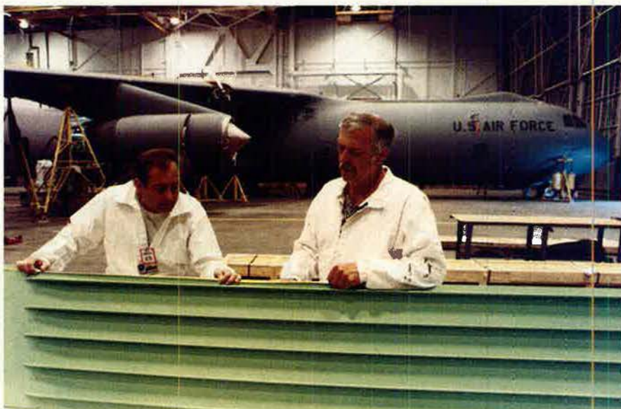
Lockheed Aeronautical Systems Co. fuel tank sealers Charles Wages (left) and Kenneth Williams measure lower wing panels for a C-141B StarLifter under repair (background). The strategic airlifters developed wing weep hole problems in 1993; 200 of 244 C-141s have been returned to service.
