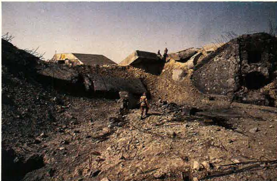
A damaged hangar at Ali Al Salem AB, Kuwait, shows the devastating effect of the 750-pound M117 bombs, which had psychological effects as well. Twenty to forty percent of Iraqi deserters mentioned the B-52s' ground-shaking bomb runs.
