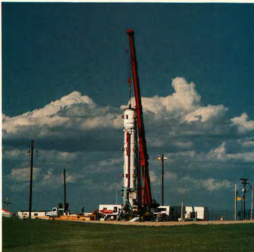
Out on the western Great Plains, ICBM modernization is becoming a reality. Pictured here is installation of a canister containing an LGM-118 Peacekeeper component at F. E. Warren AFB, Wyo. The first fifty Peacekeepers will be in place this year.
