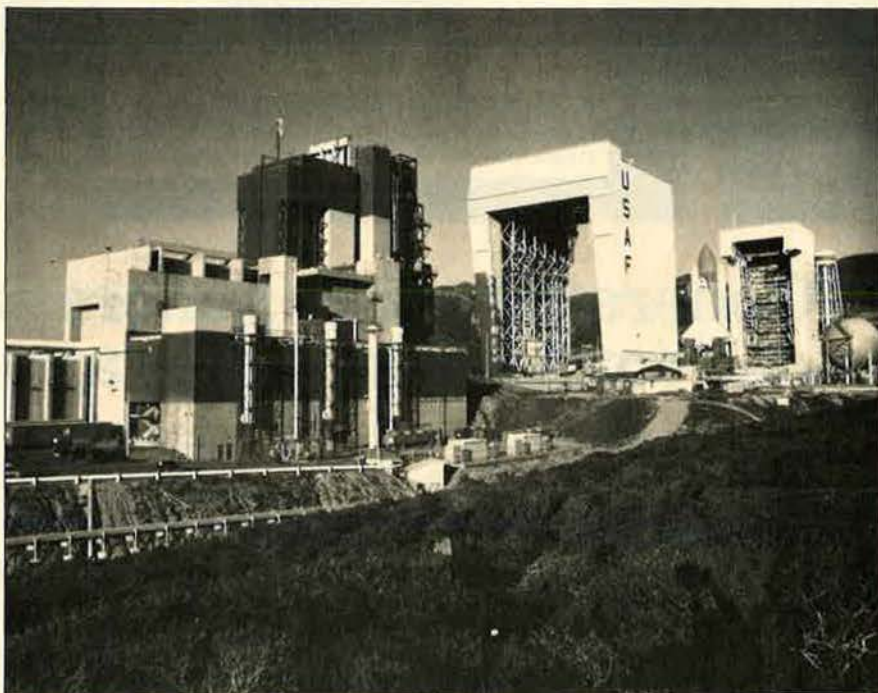
Giant, movable buildings will prepare the Space Shuttle for its first launch from Vandenberg AFB, Calif. From left are the payload and changeout facilities, the Shuttle assembly building, and the service tower. The Enterprise is at rear.
