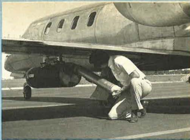
Above: Special missions Learjet 35A, with Hayes International TGX-1 visually-augmented target under starboard wing and Interdyne Corporation LJ-25 sonobuoy/flare dispenser under port wing. Right: Loading LUU-2B flares into the Learjet's LJ-25 dispenser
