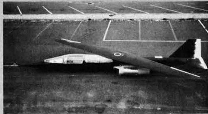
The NASA Ames AD-1 oblique-wing research aircraft, nearing completion in January 1979. These photographs show it with the wing in conventional and skewed positions
