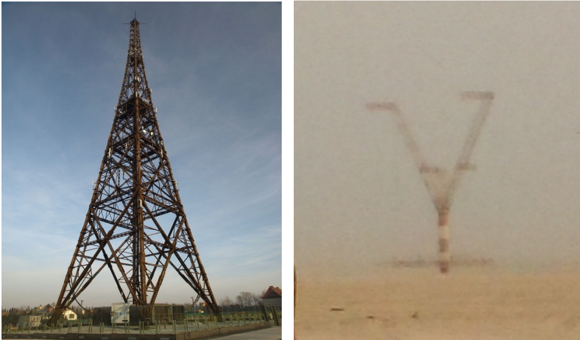
Figure 11. The left image shows a “typical” tower, wide at the bottom and narrow at the top. The right image shows the “Y” tower located north of the tower array.
