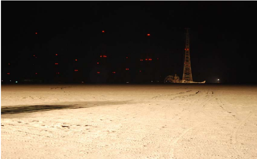
Figure 5. An image of tower lights at night with one to two red lights on top and two to four red lights midway up the tower (photographed on 5 April 2012)
