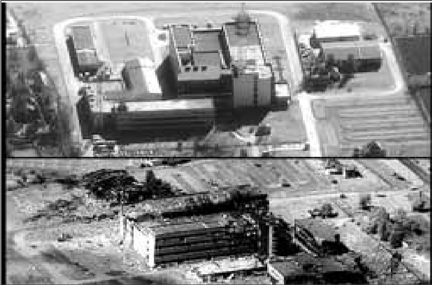
Now, the BDA. The photo at left shows prestrike and poststrike conditions of the Serb radio relay and TV broadcast site at Novi Sad. Below, the photo demonstrates the devastation of the Ponikve Airfield in Serbia by multiple bombs; they have cut the runway and taxiways several times.
