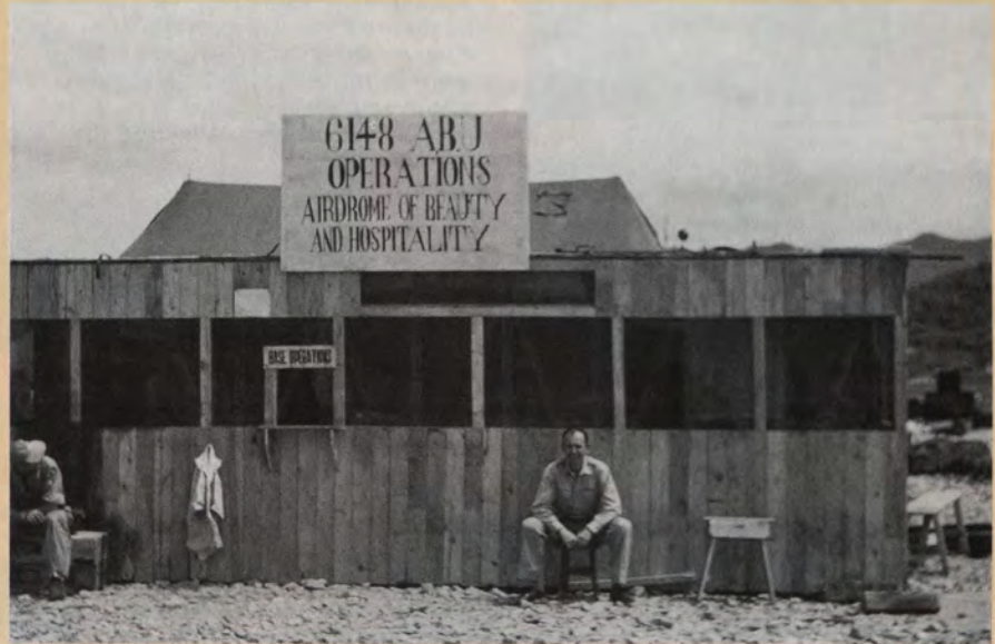
The transient aircraft commander waiting patiently for approval of his flight clearance is Maj. Russell E. Dougherty. The scene is the newly constructed Base Operations Building at Pusan AB (K-1), South Korea. The Major went on to become commander in chief of Strategic Air Command and (from 1980 to 1986) Executive Director of the Air Force Association. General Dougherty, USAF (Ret.), lives in Arlington, Va.
