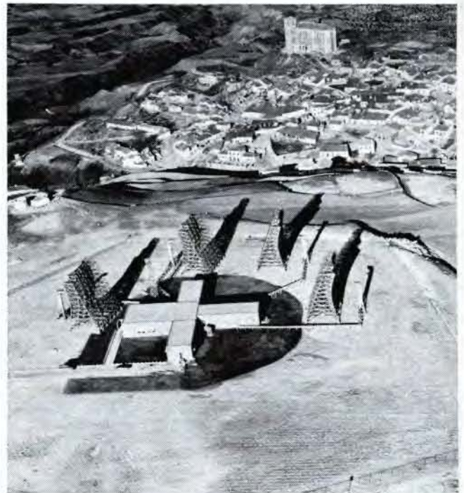
This Communications Service troposcatter antenna array near Humosa, Spain, is one of a number of AFCS stations which provide multichannel voice and teletype service for Air Force operations in Western Europe, stretching from England through Spain across Mediterranean to North Africa.
