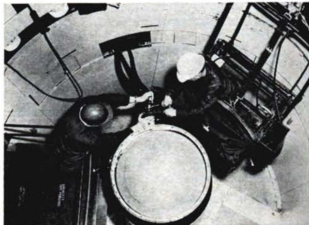
Realism is the theme in ATC's training, as witness this scene at Chanute AFB. Two ATC students are learning the delicate job of attaching umbilical cord to Minuteman ICBM as it sits in silo. Cord feeds computer data to missile.
