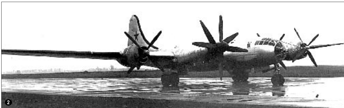
[1] This is the Myasishchev Experimental Design Bureau ramp in the 1950s, with a Tu-4 Bull in foreground. The Tu-4 first flew in 1947. This aircraft was converted in 1952 into a flying laboratory to test a landing gear for the M-4 Bison bomber, seen on the taxiway. [2] A Tu-4LL outfitted with an eight-bladed propeller and an NK-12 engine for the Tupolev Tu-95 Bear strategic bomber. The then-new power plant was tested at Ramenskoye in 1952. [3] In 1951, this Tu-4KS was used as a test-launch platform for the KS missile, designed by Mikoyan. The missile went operational on Tu-16KS Badgers in 1957. [4] Mikoyan's MiG-9 took to the air for the first time on April 24, 1946, about three hours before the Yak-15. [5] This prototype Yak-15 was extensively tested in taxi and wind tunnel trials at Ramenskoye. The fighter was designed in the 1940s, and based on the Yak-3. The engines were based on a German engine. Yakovlev pulled the piston engine from its Yak-3 and replaced it with a jet engine.
