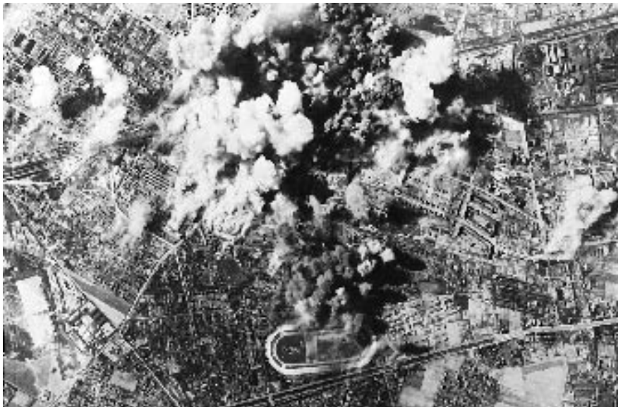
Smoke plumes rise in the aftermath of a B-17 raid on the Daimler-Benz tank works, Berlin, in March 1945.
