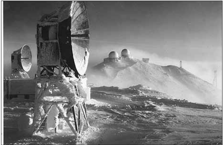
On the ground in the late 1950s, air defense in the far north included radars on the DEW Line, amid windswept peaks on the frozen landscape. Construction of the DEW Line was the largest building project in the Arctic.
