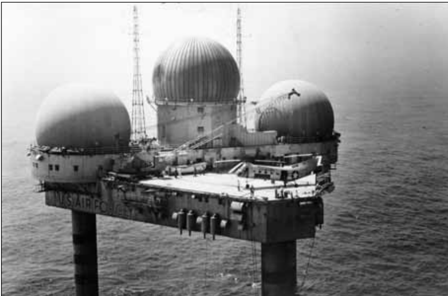
A more radical idea for early warning: Texas Towers, named for their resemblance to oil-drilling platforms. The radar stations rose from the sea, off the northeast coast of the US. This is TT-3, located south of Nantucket, Mass. The last of the towers was decommissioned in 1963.
