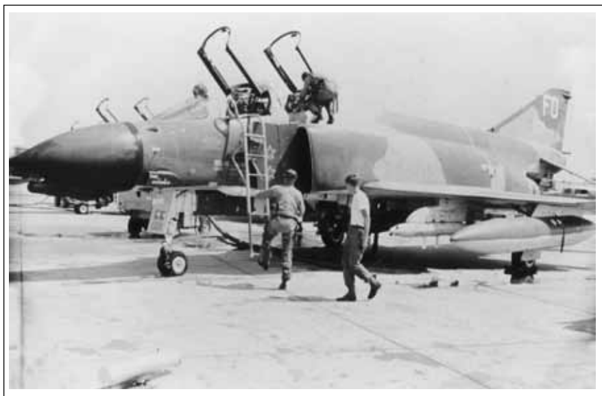
This version of the F-4 participated in Operation Bolo. Note its inboard pylon ECM pod. The F-4’s initial lack of an internal gun put it at a disadvantage in a close-in fight, but this one’s two red stars indicate success over enemy MiGs.
